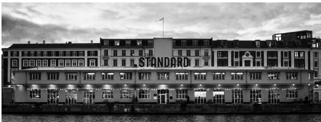
The name of Copenhagen's new jazz club, The Standard, pays tribute to the history of its Art Deco building which Danish architect and Royal Building Inspector Kristoffer Nyrop Varming designed in 1937 in the midst of the golden age of timeless "standards" composed by George Gershwin, Cole Porter and others. Photo courtesy of en.thestandardcph.dk.
