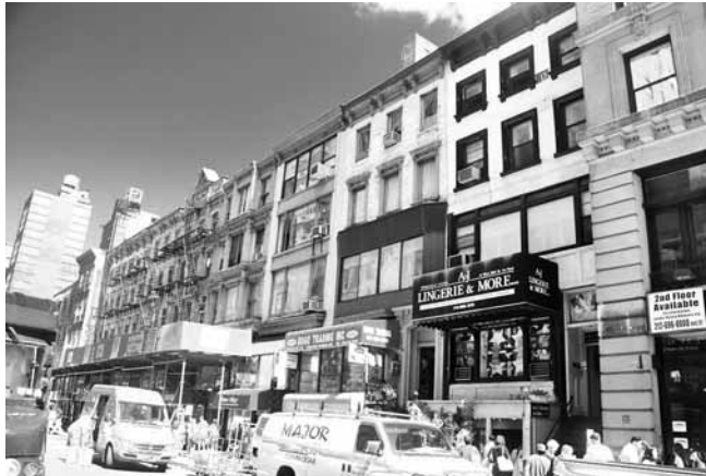
These painted-over brownstones at 55 to 41 West 28th Street, Manhattan, housed America's first sheet music industry.
